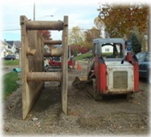
Trench Box used to shore up the sides of a dig.
