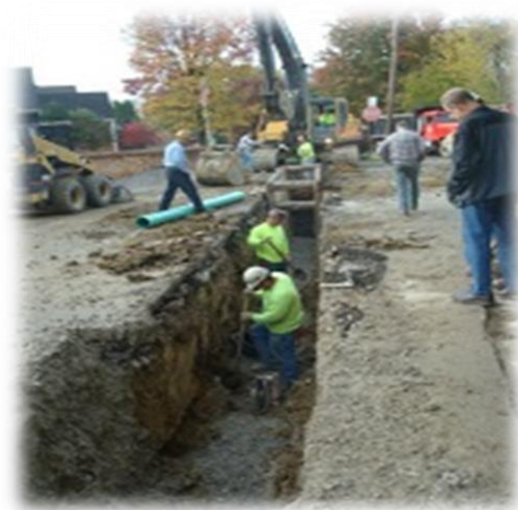
Sewer lines replacement
