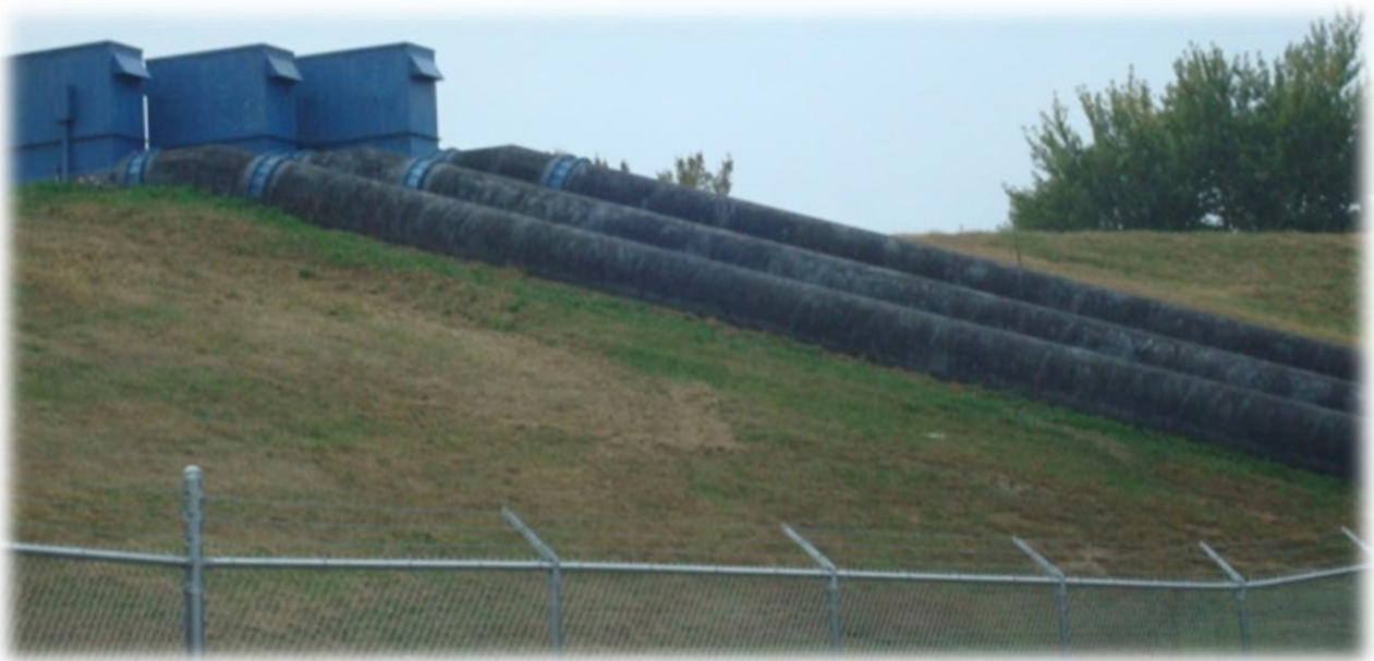
Discharge Pipes – Pumps off flood water
