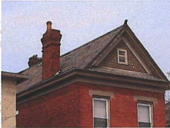
Example of a well maintained chimney on a historic building
