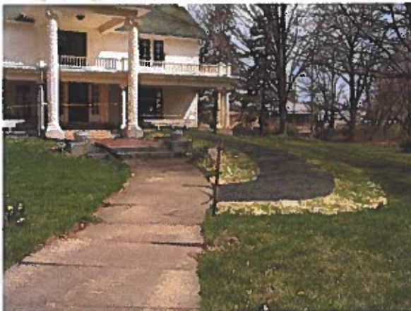
Grass pavers create a ramp without concrete and without altering the historic entrance to the building.
