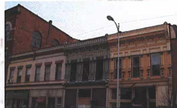
A good example of upper floor windows that are rhythmic.
