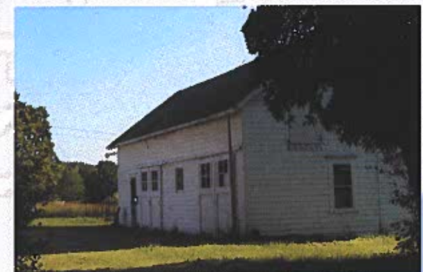
Example of outbuilding that has not been properly maintained.
