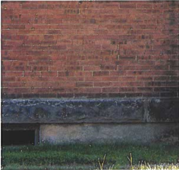
A good example of a historic foundation.
