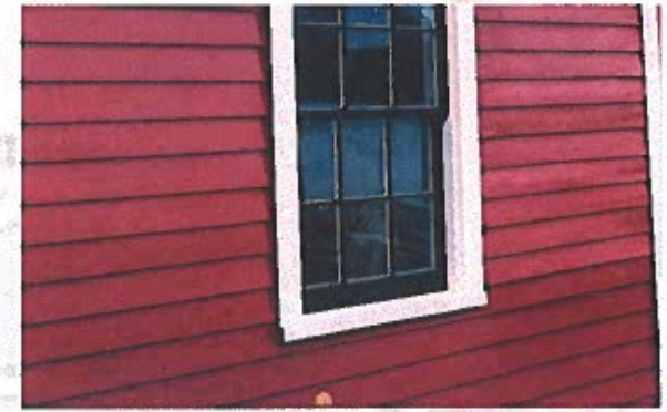
A good example of new siding matching historic siding.
