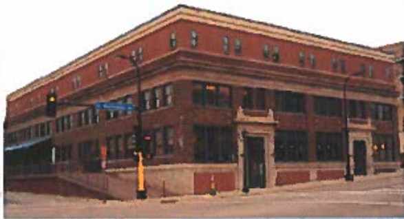
Example of an inappropriate addition to the roof of an existing structure.
