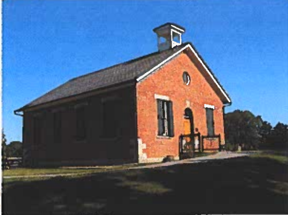
Land was graded and a sloped sidewalk installed to create a gentle ramp that makes the building accessible without destroying the appearance.
